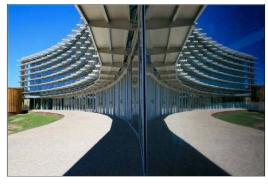
The Applied Research and Development facility at NAU has an exposed frame of concrete, which stores thermal energy and provides 50 percent of the building's heating requirements. (Northern Arizona University)
